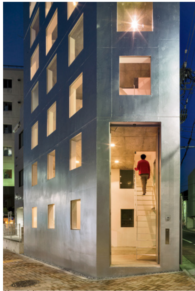
View of the entry and site pavers from the northeast.
