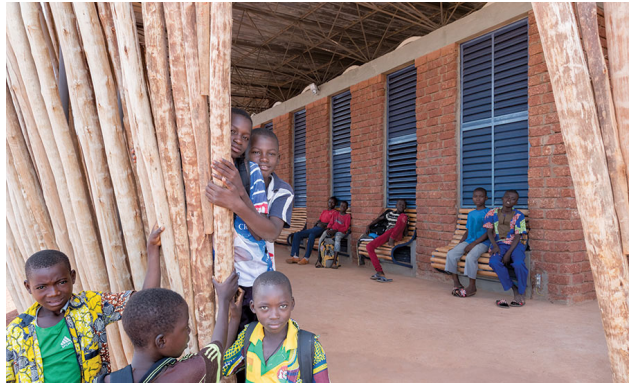
Between the eucalyptus-wood screen and the brick walls of the school's rectangular modules is a sheltered space where students can socialize.
