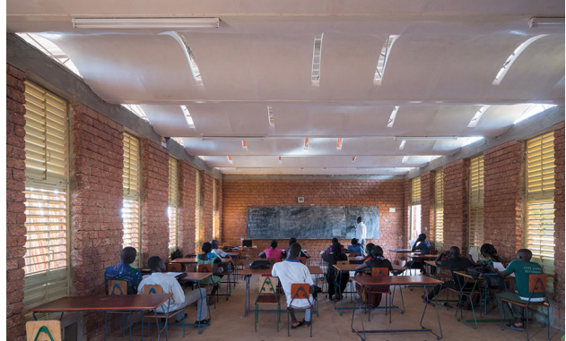
Undulating Classroom ceilings are made of gypsum fiberboard, straw, and cement mortar. Slits in these surfaces admit diffuse daylight.
