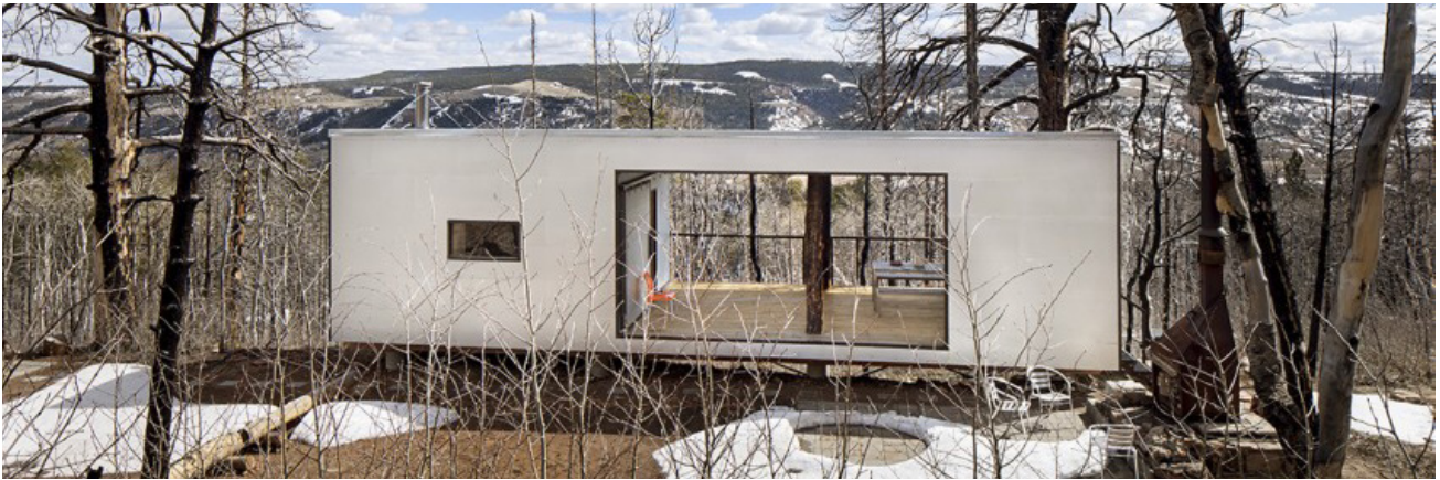
North elevation showing sole tiny window to enclosed space.
