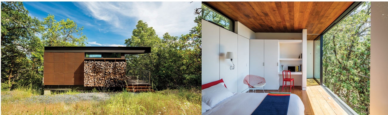
Cabin 2 viewed from the southwest and its interior showing operable window wall and clerestory.
