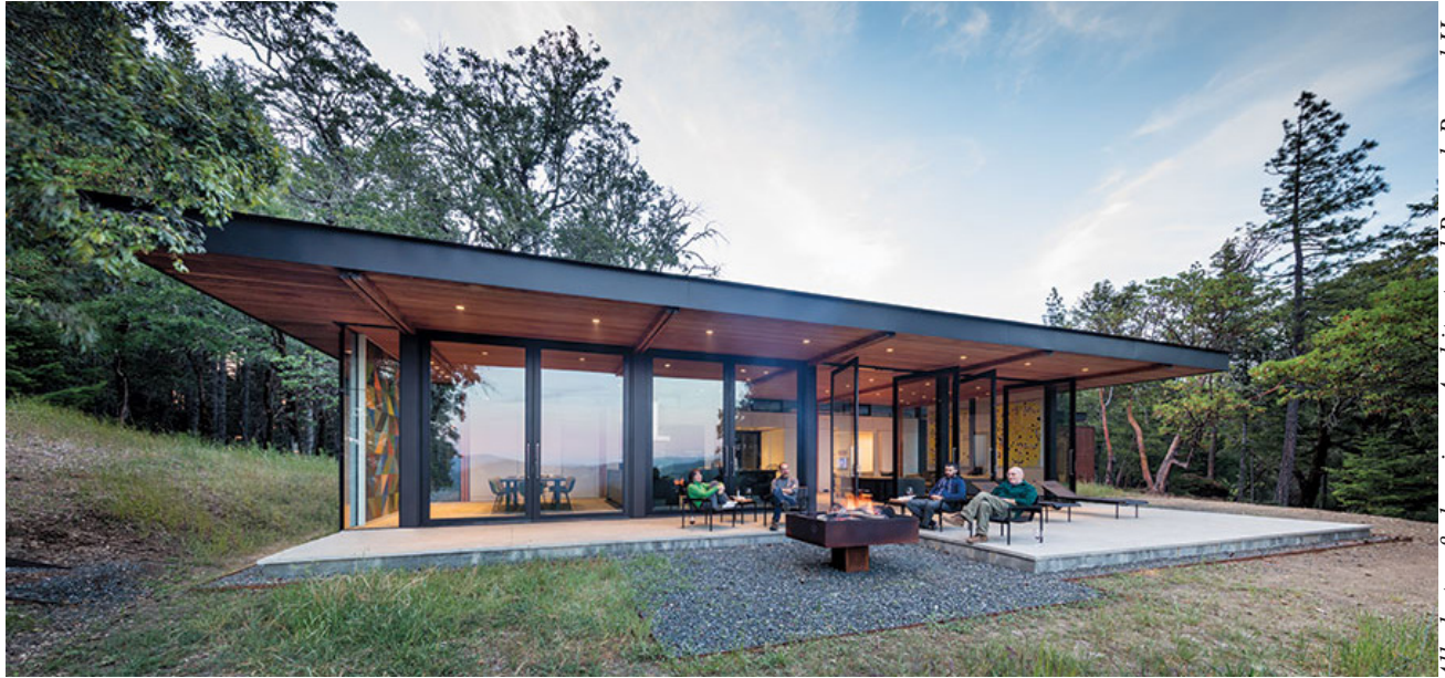
The southeast-facing wall is composed of pivoting glass doors that open to the living dining kitchen area.
