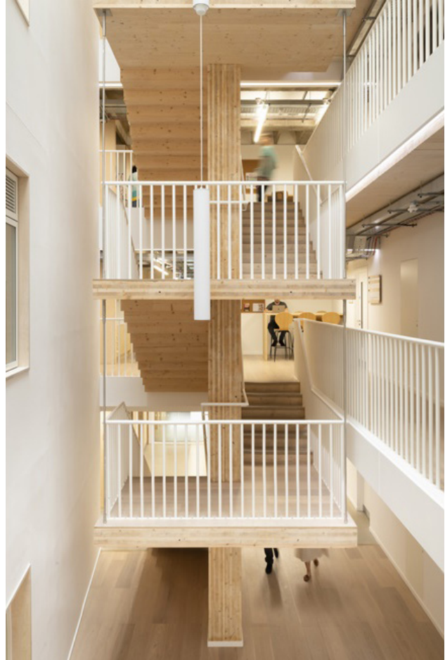
Atrium view of the CLT cantilevered stair with LED lighting fixture in the foreground.
