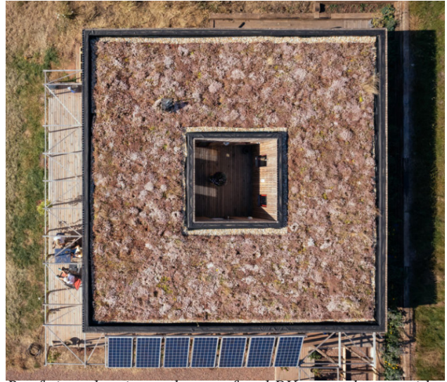
Roof view showing sedum roof and PV array that provides 22% of the electricity required.
