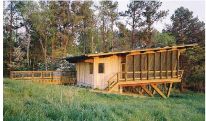
The Ecostation, viewed from the northwest, perched above the prairie, is accessible by a bridge that passes alongside its rainwater cistern. The deck on the south side has a commanding view, spoiled only by a nearby interstate highway.
