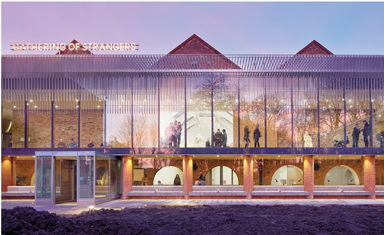
Above: Garden view of the fully glazed Promenade Gallery with the Central Exhibition Gallery visible in the background.
