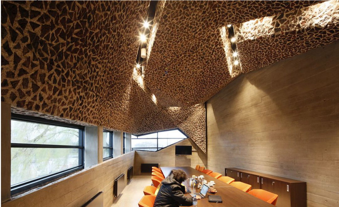
Conference room with board-formed concrete walls and picado ceiling
