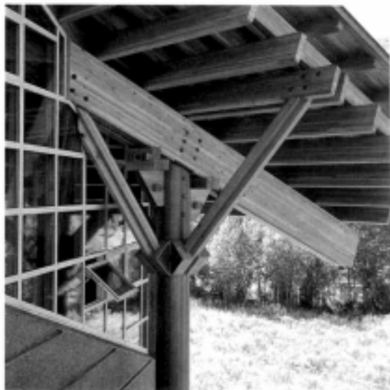
An operable north-side living room window protected by the overhanging roof.
