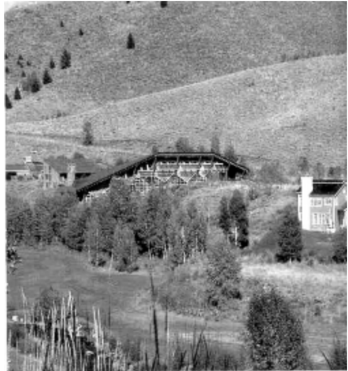
View of the south facade..
