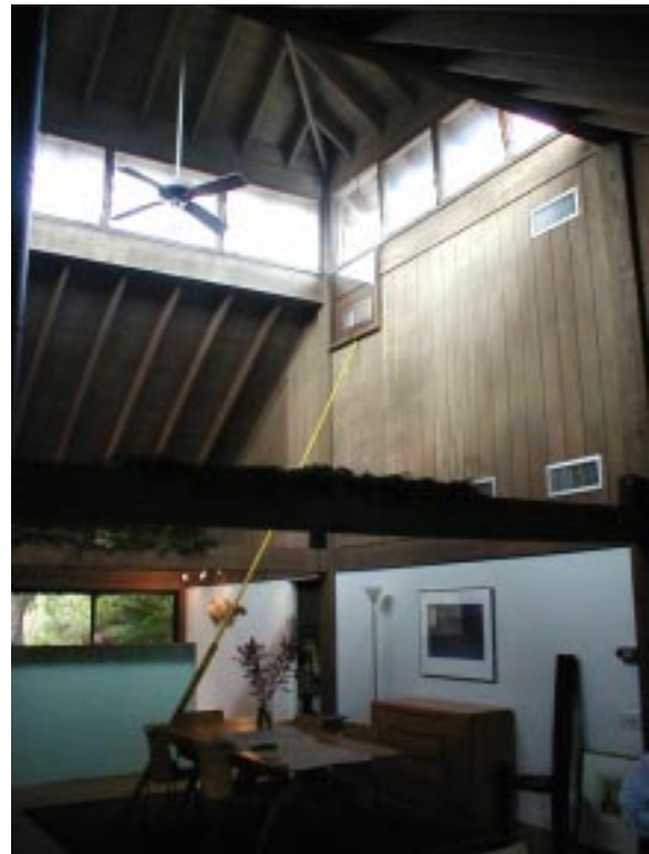
Main room with belvedere windows, ceiling fan and pole for window operation.
