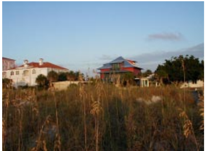
An early twentieth century cracker house on the Gulf coast.
