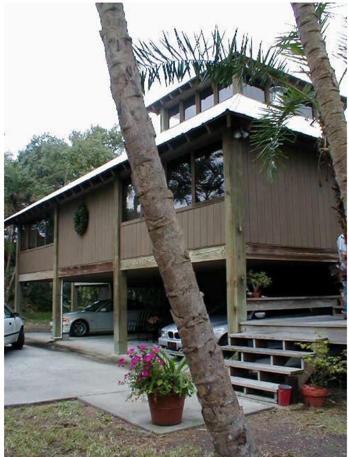
SE corner showing belvedere and stairs to deck.
