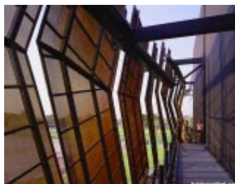
The wire screen is held away from the building and provides filtered shade from the morning sun.
