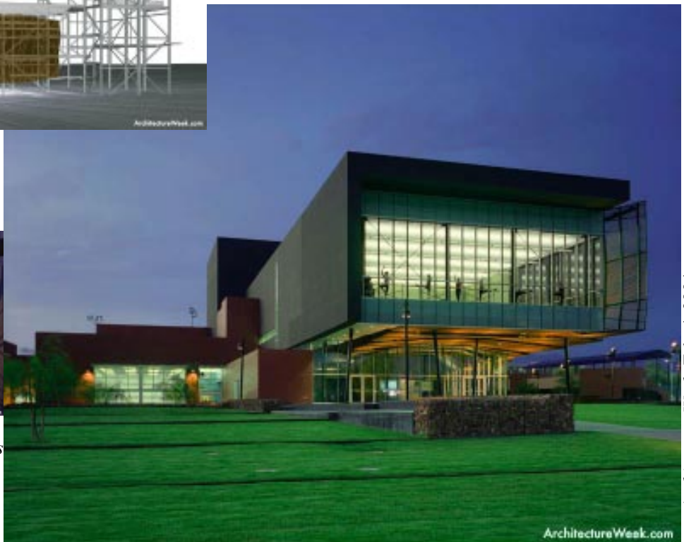
Seen from the southwest, the second floor dance studio seems to cantilever over the landscape .
