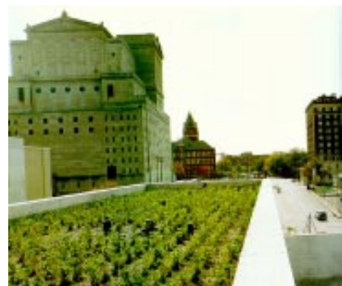
The office wing has a green roof.
