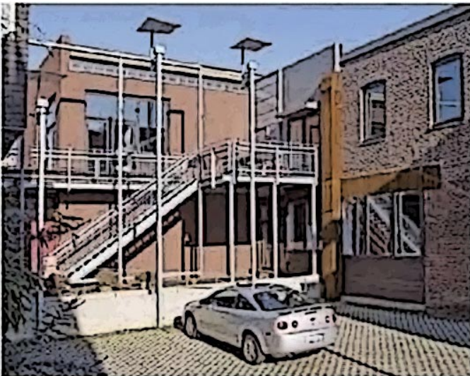
View from the parking court toward the northeast.
