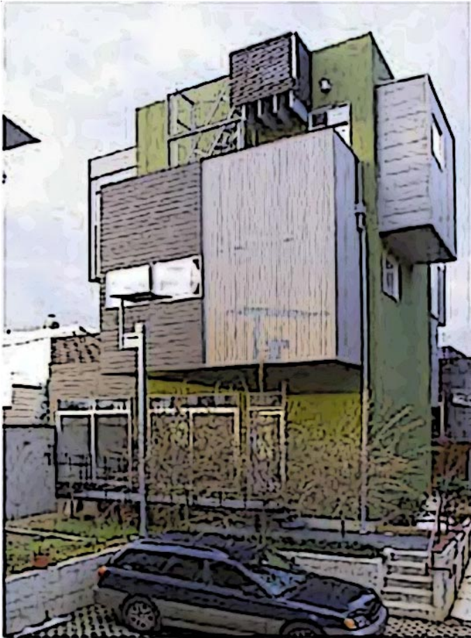
Northeast facade of one of the trinities from the parking court.
