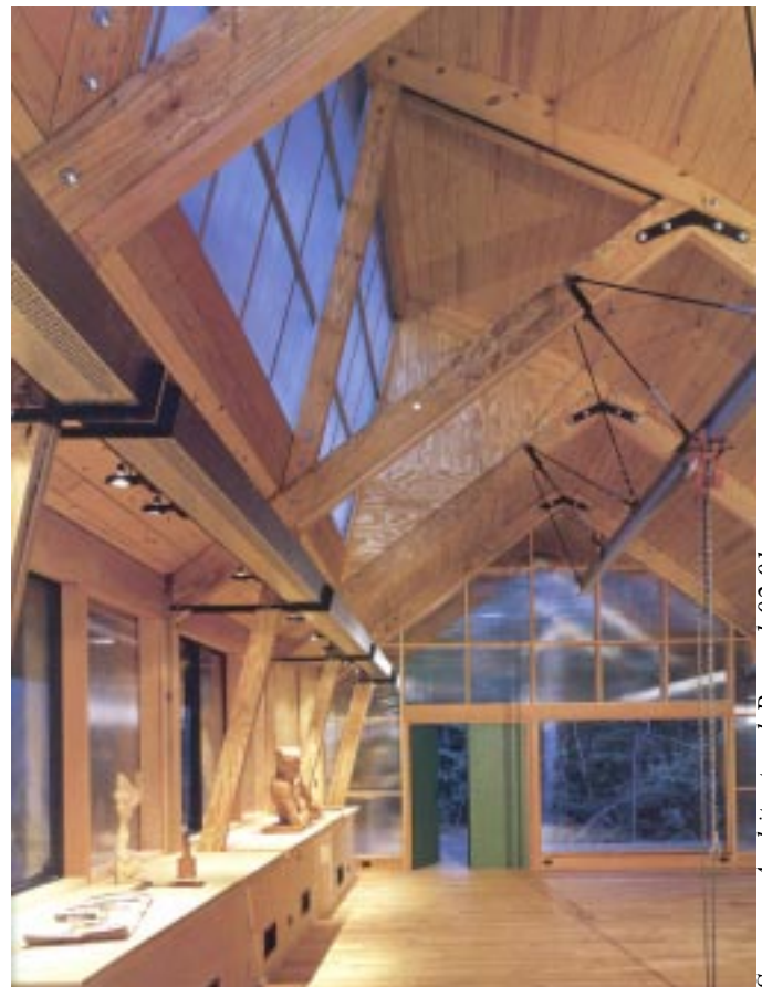
Interior view looking east.
