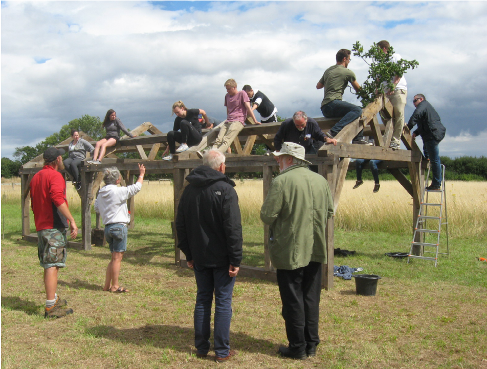
Students constructing a heavy timber frame in Alison and Rupert's field in 2017.
