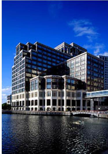
25 Cabot Square Skidmore Owings & Merrill. ( www.canarywharf.com )
