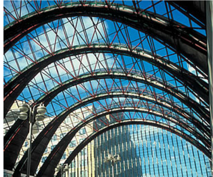
Canary Wharf Docklands Light Rail Station - ( www.ucl.ac.uk )
