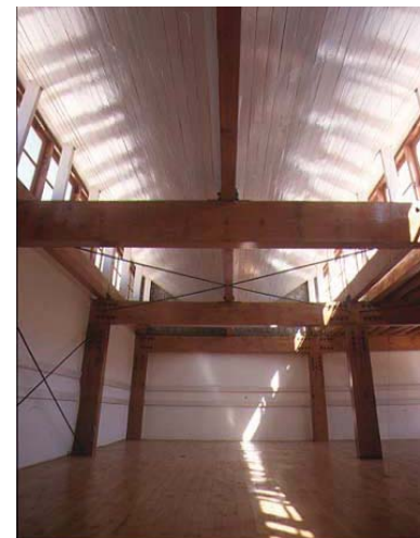
4.10 The splayed roof acts as an indirect daylight source in the classroom. Note lack of electric lighting fixtures.
