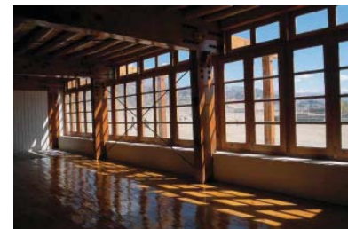
4.07 School rooms feature southeast-facing direct gain windows that ensure early morning warm-up in Shey's sunny climate.
