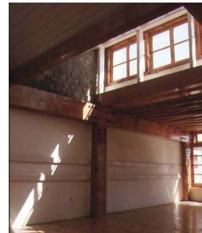
4.09 Clerestory and view windows provide daylight to the classrooms.
