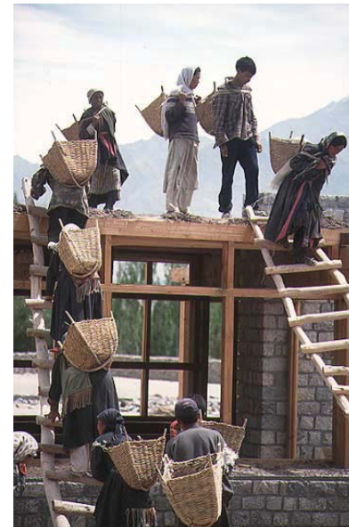
4.14 Arup worked with local construction crews.
