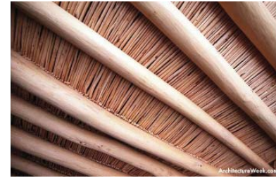
4.13 Roof construction uses local poplar rafters and willow sheathing.
