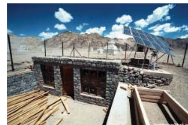
4.12 The pumphouse at the wellhead is powered by a sun-tracking PV array.
