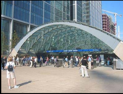
Canary Wharf Underground Station Source: http://www.mykreeve.net/london/docklands/canary_wharf_tube_station.jpg
