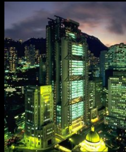
Hong Kong Bank Headquarters, Hong Kong Source: http://www.fosterandpartners.com/
