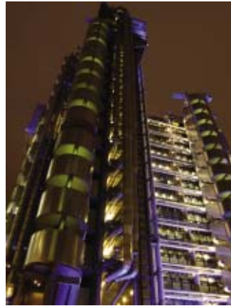
The Lloyd's Building
