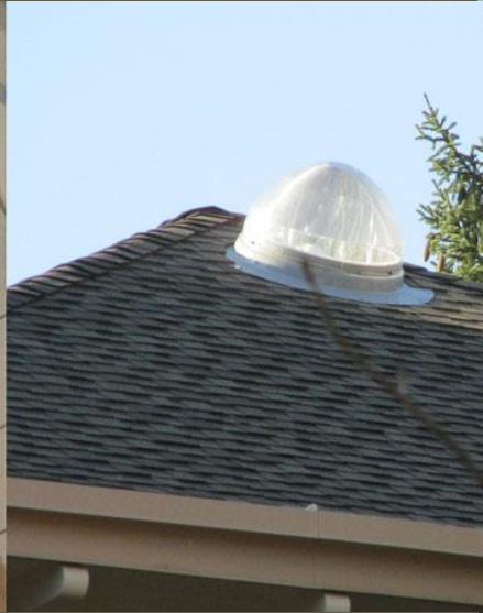
Fall term Solatube installation
