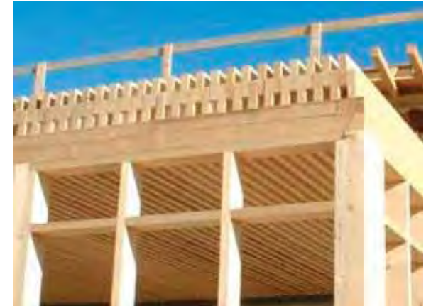
D-Dalle Timber Slab
