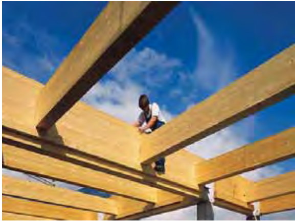
Glulam Timber Framing
