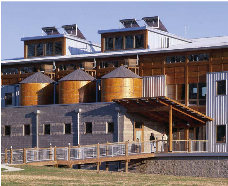
Chesapeake Bay Foundation Rainwater Catchment System
