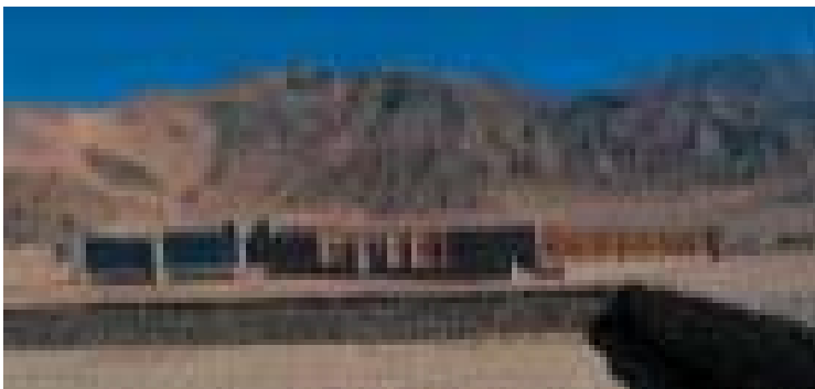
5.5 The Druk White Lotus School classrooms appear to emerge from the landscape. Their orientation takes advantage of early morning solar access.
