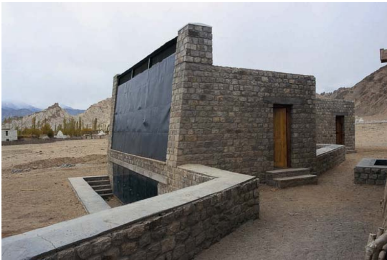
5.10 The latrine building with solar collector. CAROLINE SOHIE, ARUP PLUS ARUP ASSOCIATES
