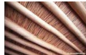
5.13 Roofs are constructed of local poplar rafters and willow sheathing. ARCHITECTUREWEEK.COM ???
