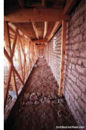
5.11 Mud brick walls are made of local materials. ARCHITECTUREWEEK.COM ???
