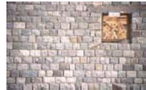
5.12 Granite block facing is stable and also locally obtained. CAROLINE SOHIE, ARUP PLUS ARUP ASSOCIATES
