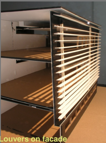
Louvers on facade
