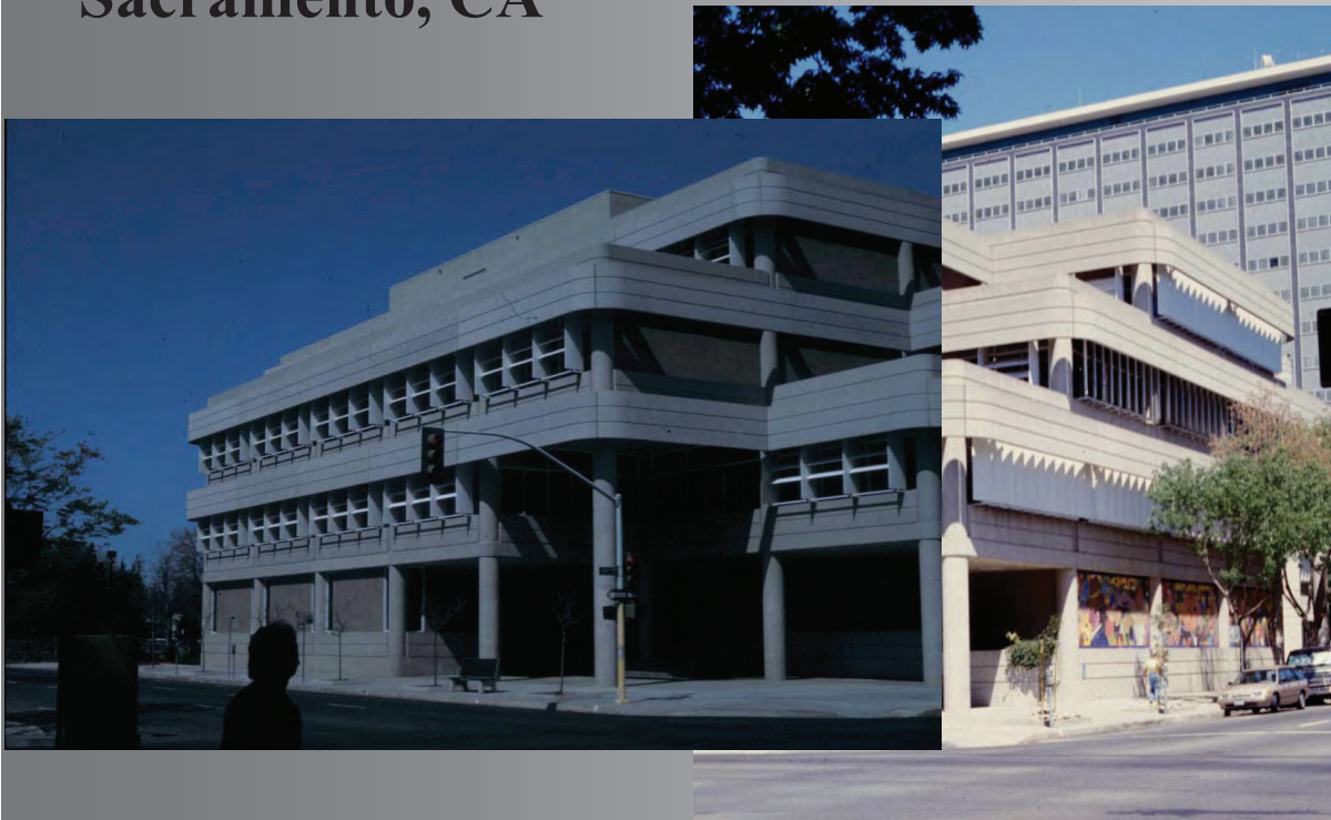
South and East facades...
