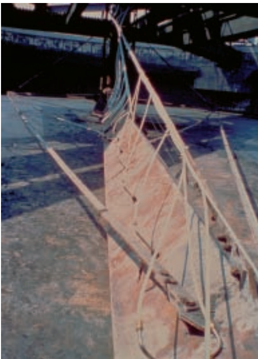
Installation of sample probes in header.
