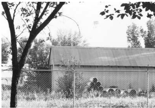
The Tin Shed, Crow Agency Photo: Frey 1974
