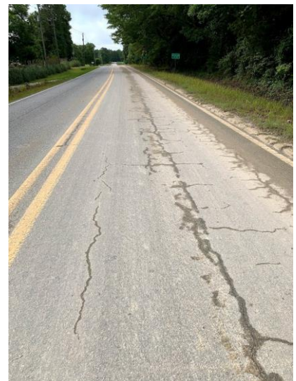
SINGLE LAYER CHIP SEAL + CRACK SEAL
