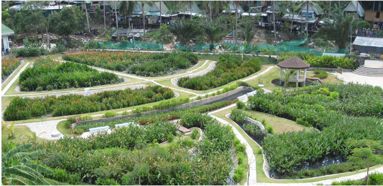
Figure 9. Koh Phi Phi Multifunctional Community Garden. Collection and distribution building far left, VSF left, HSF center, FWS right, polishing pool center (Photo courtesy Hans Brix, Aarhus University, Denmark).
